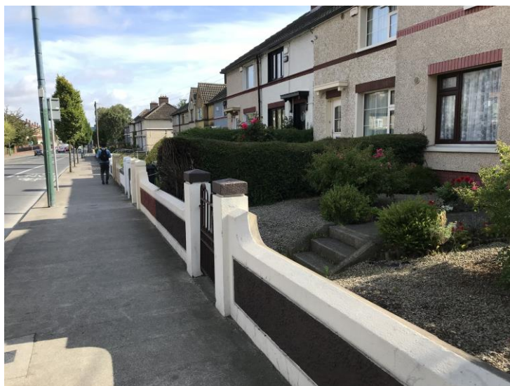
Figure 3-21: Houses on the eastern side of Harold's Cross Road north of St. Clare's School
